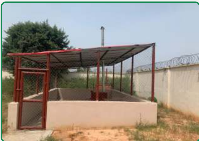
INCINERATOR AT THE YAR GAYA ISOLATION CENTRE IN KANO STATE
