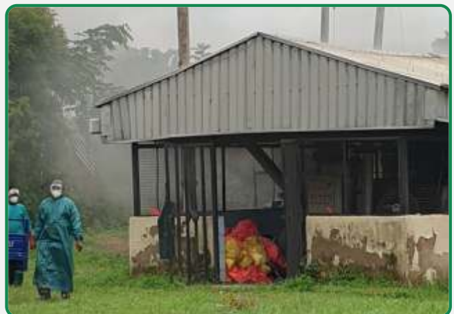
WASTE TREATMENT FACILITY AT ONE OF THE TREATMENT CENTRES VISITED AND ASSESSED BY THE SAFEGUARDS TEAM
