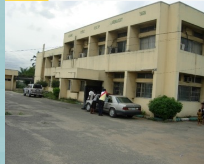
CPHL before renovation
