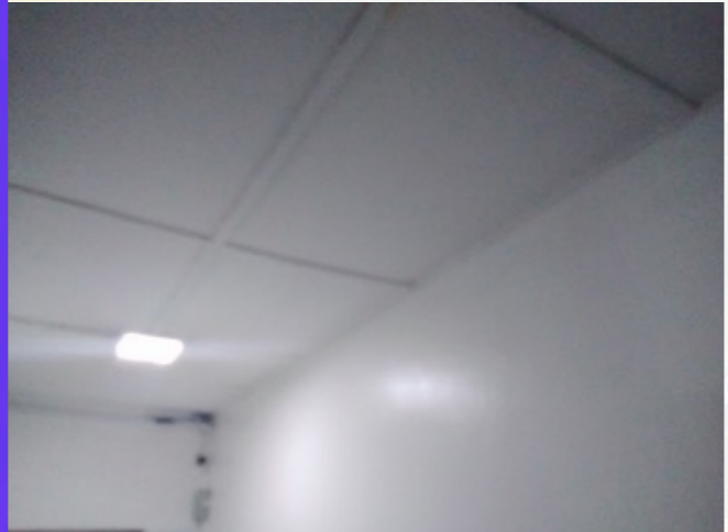
The ceiling of the laboratory passage after renovation
