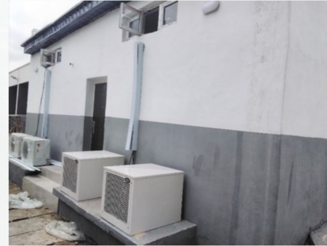
Construction of cold room for cold chain management.
