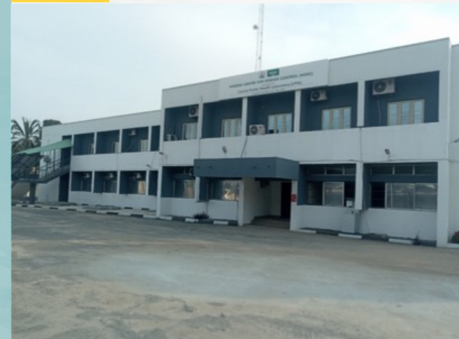
CPHL after renovation
