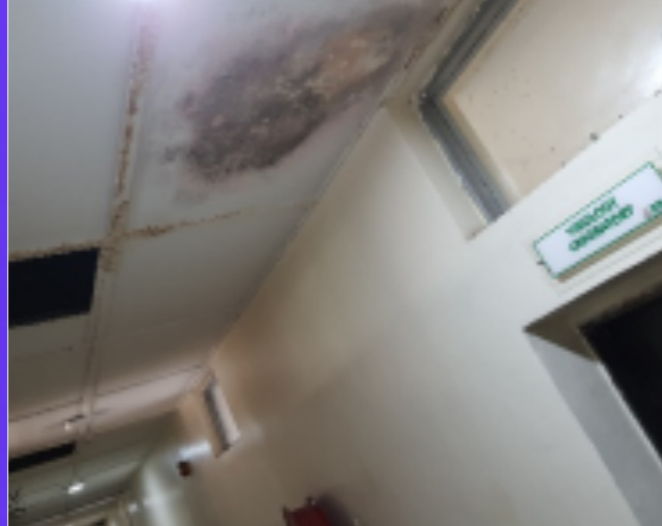
The ceiling of the laboratory passage before renovation
