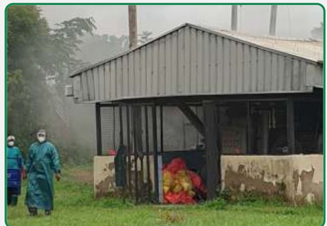
WASTE TREATMENT FACILITY AT ONE OF THE TREATMENT CENTRES VISITED AND ASSESSED BY THE SAFEGUARDS TEAM
